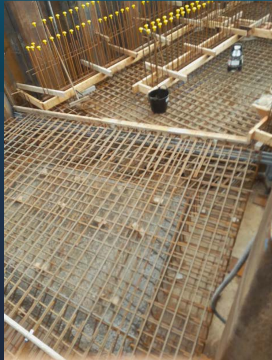
Installation of rebar and formwork at kicker level 'cont'
