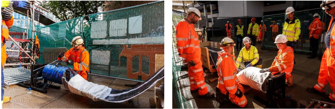
Figure 6 – Mounting of liner and burst bag to end cans.
