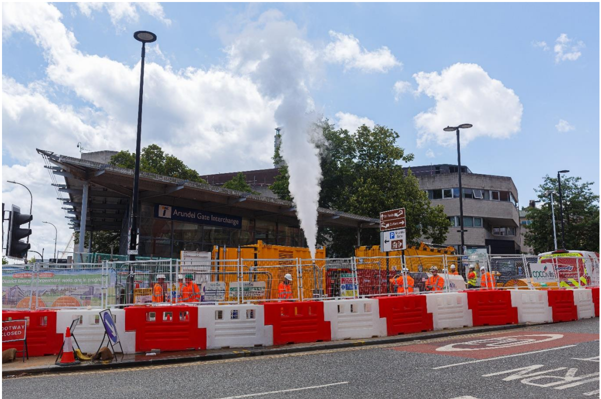
Figure 12 – Completion of the lining works and releasing of steam pressure.
