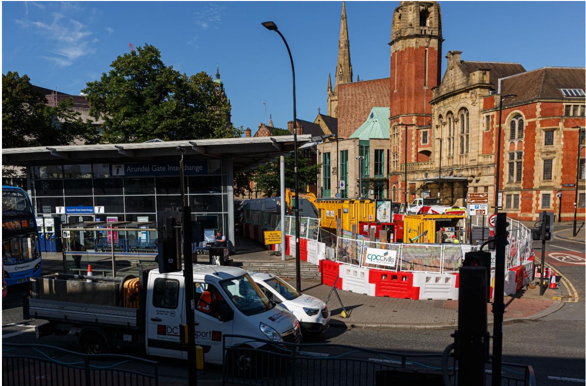
Figure 11 – Site Set Up.
